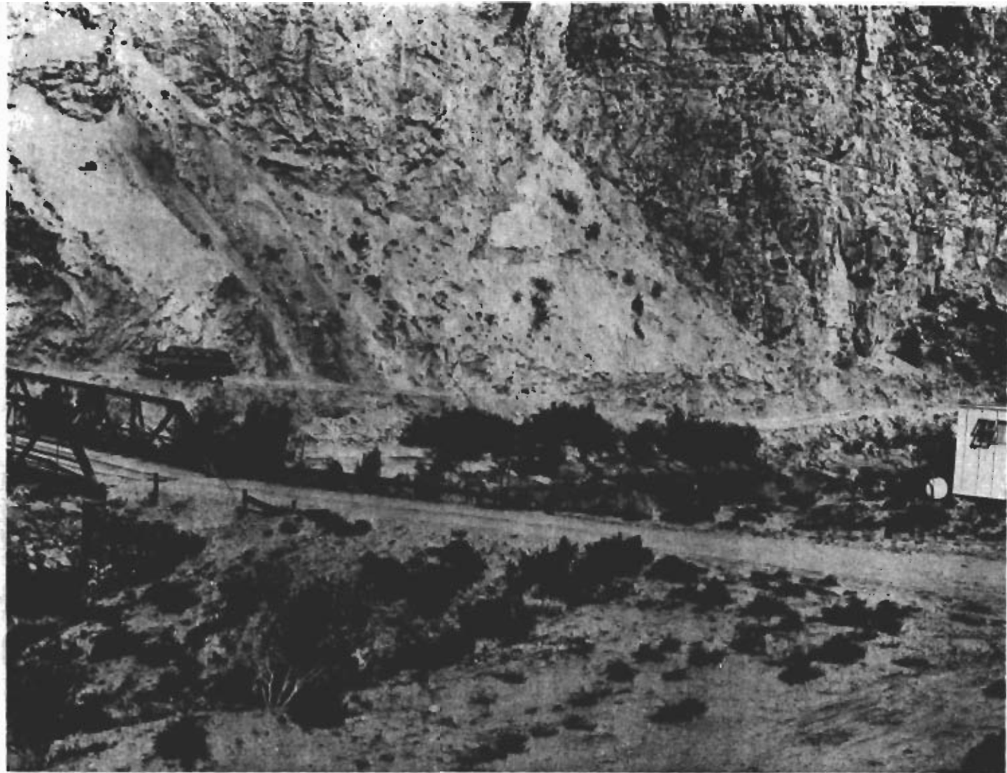
LaVerkin Springs Unit - view of lower control damsite.
