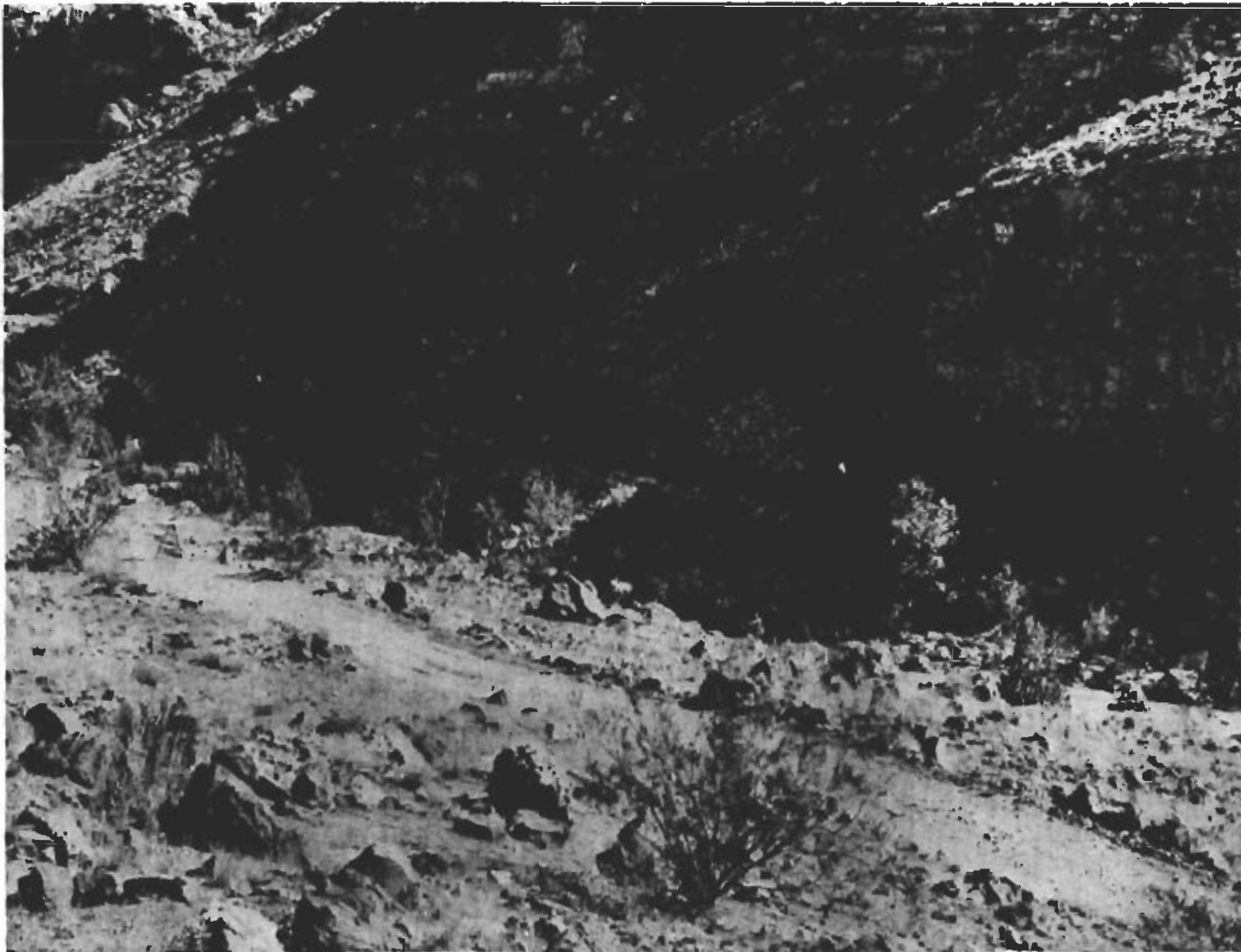
LaVerkin Springs Unit - view of upper diversion damsite.
