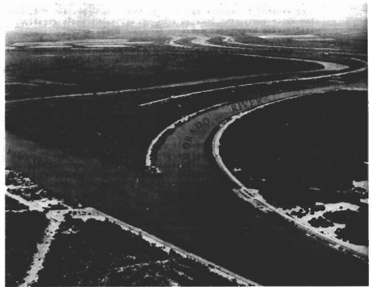
Return flow utilization - view of Palo Verde outfall drain.
