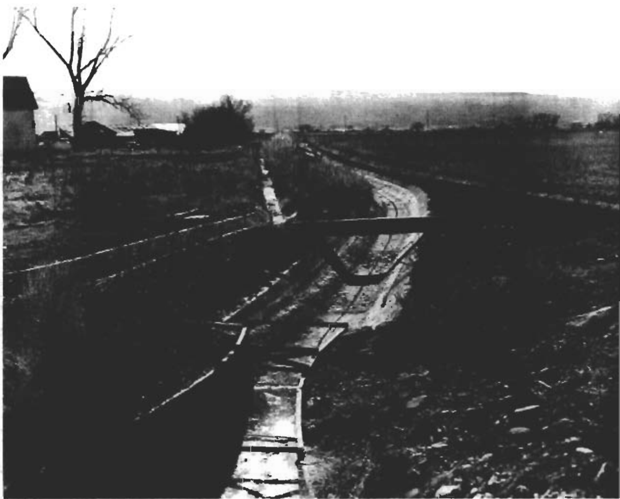
Grand Valley Basin Unit, concrete-lined lateral.
